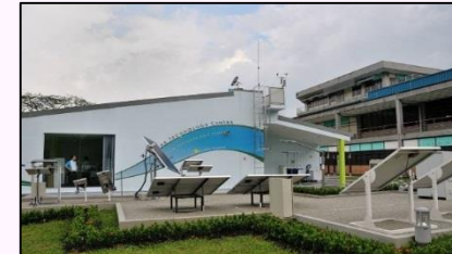
Solar Technology Centre
